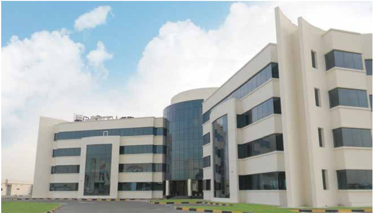
Pacific Control's new Data Centre Campus
